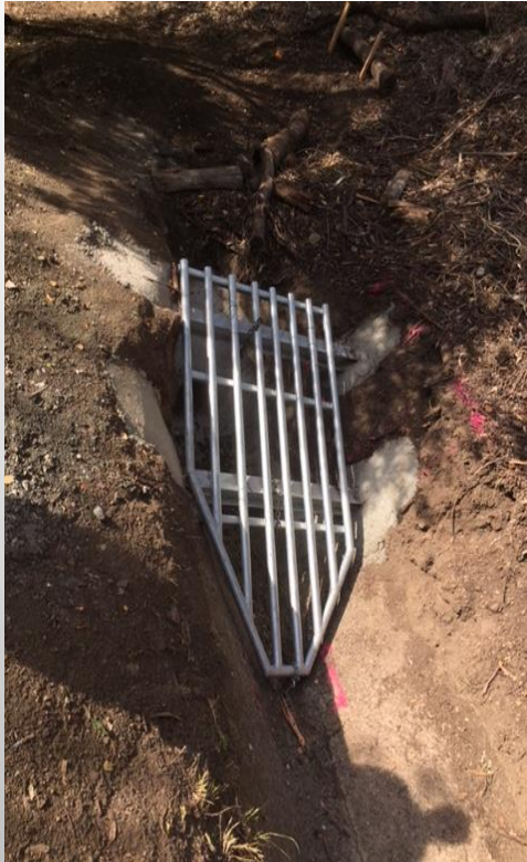
HILGARD CULVERT TRASH RACK
