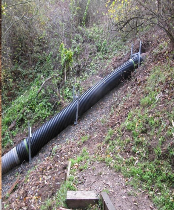
PARK HILLS CULVERT
