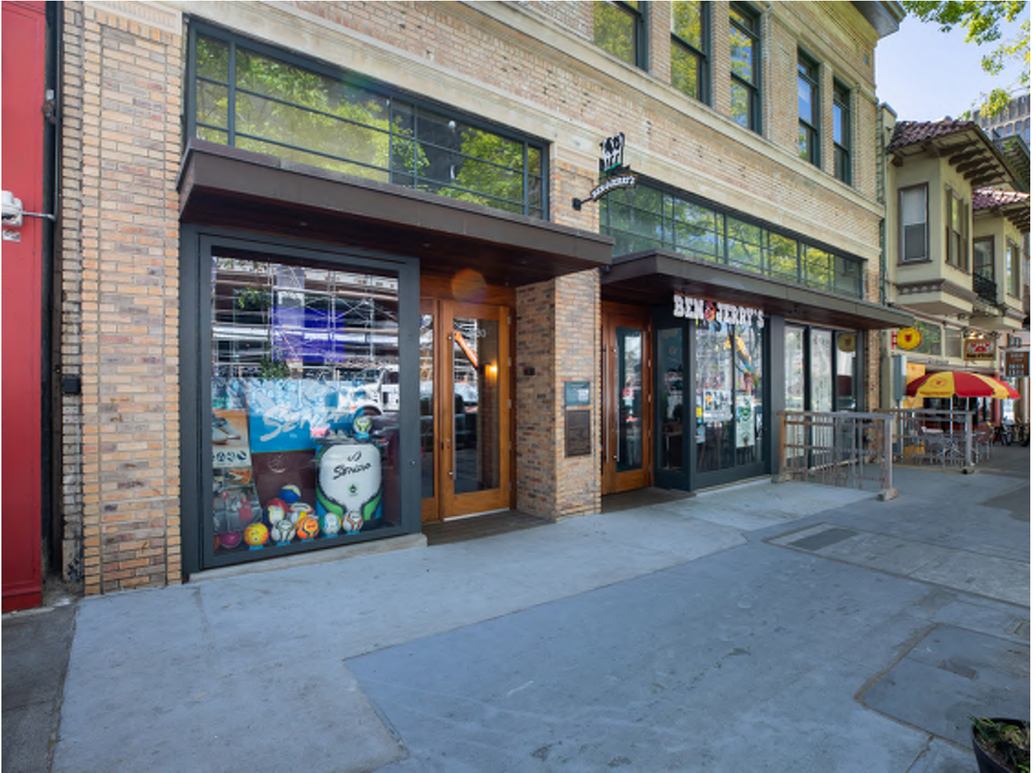
VIEW FROM CENTER ST SIDEWALK LOOKING WEST
