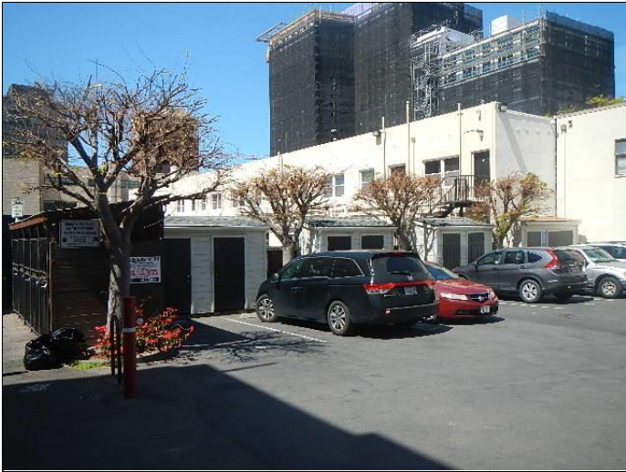
22. Storage shed behind 2128 building
