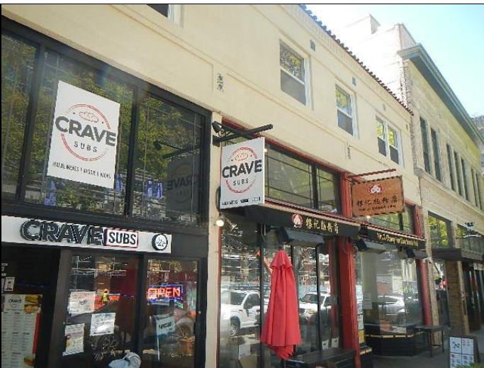
5. North façade of 2142 building
