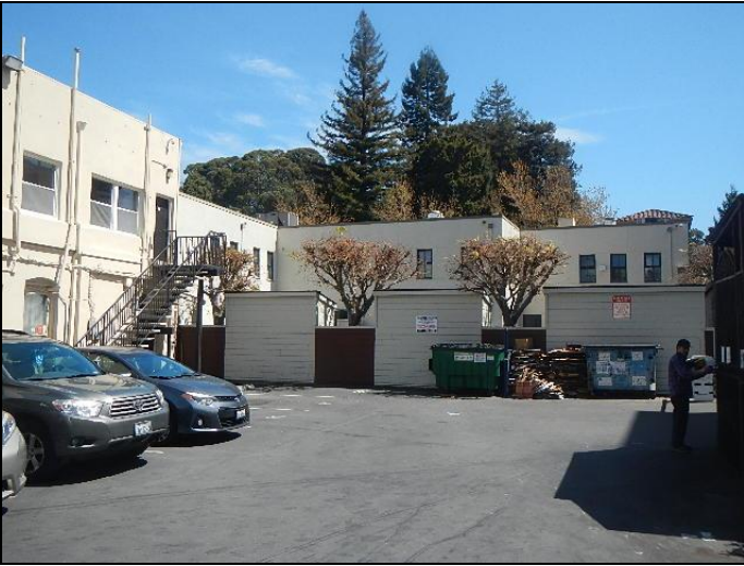
1. Parking and rear façade of 2128 building
