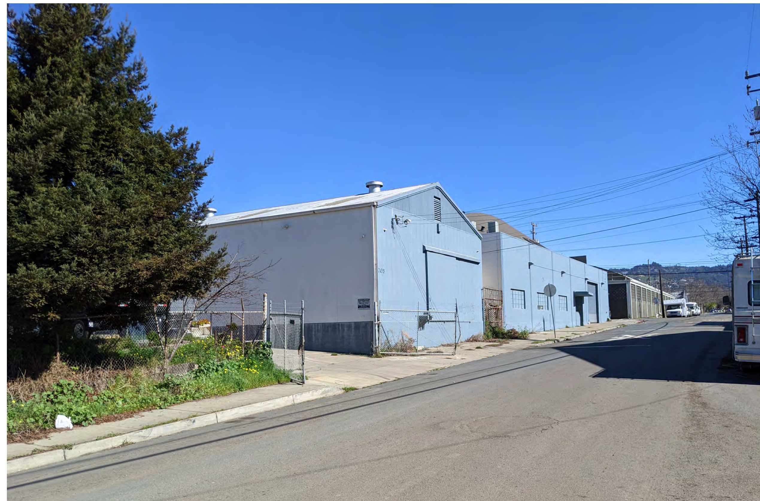
VIEW FROM BANCROFT WAY: EXISTING - 2
