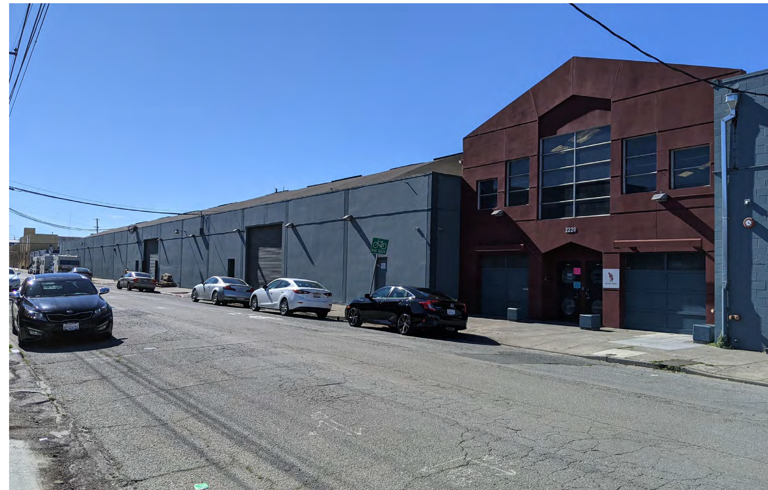
VIEW FROM 4TH STREET: EXISTING - 1
