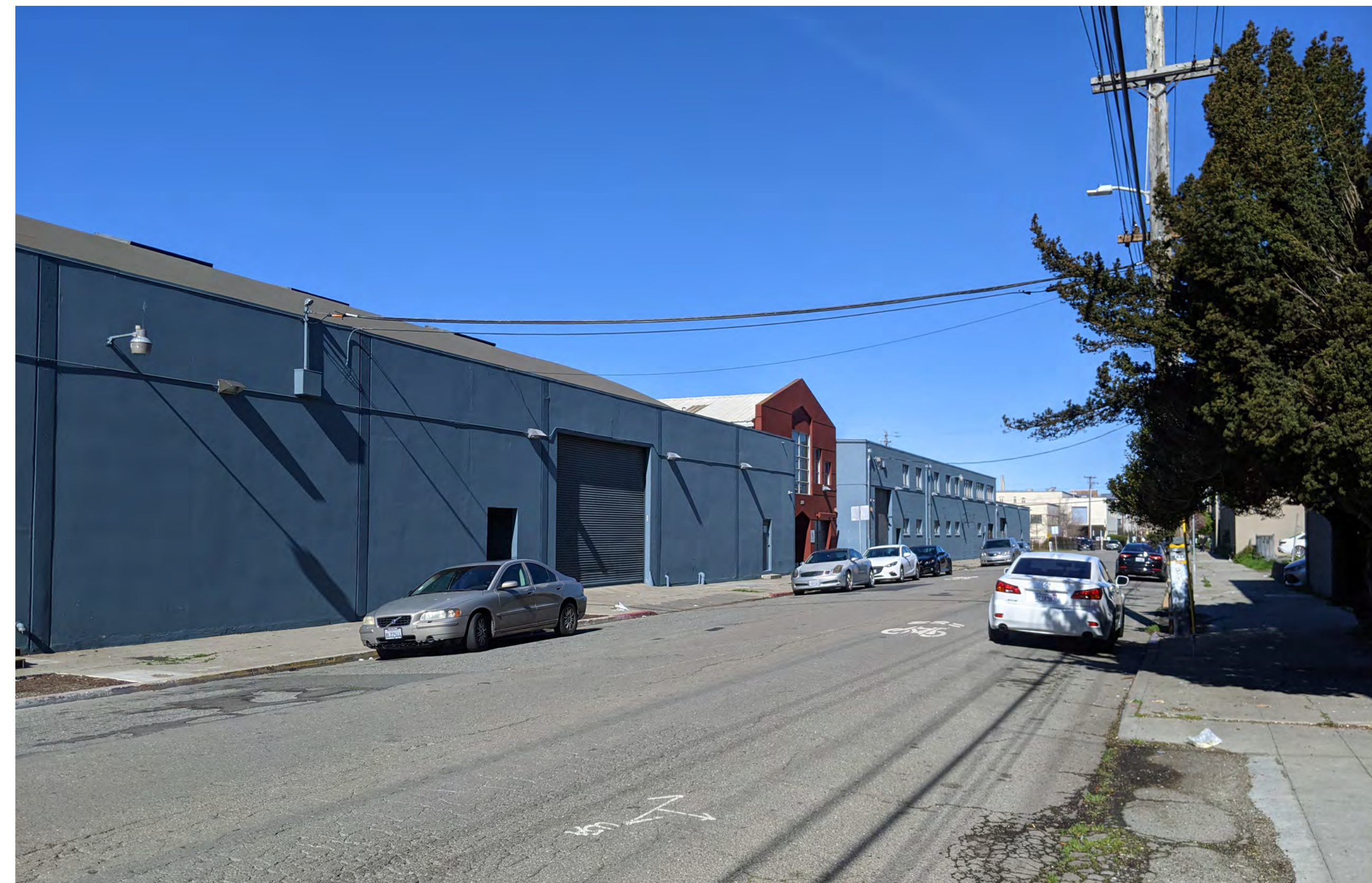
VIEW FROM 4TH STREET: EXISTING - 1
