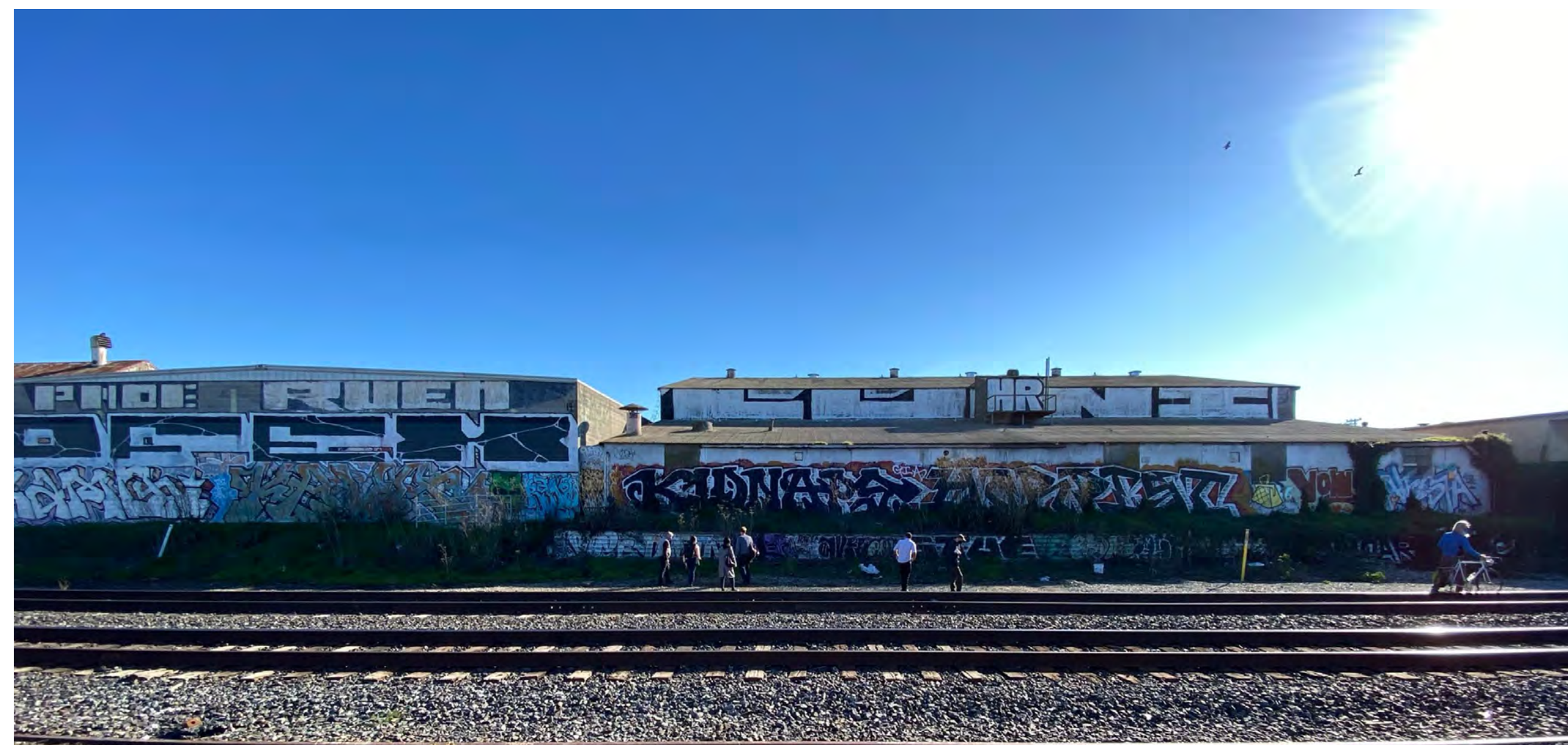
VIEW FROM RAILROAD CROSSING: EXISTING - 1
