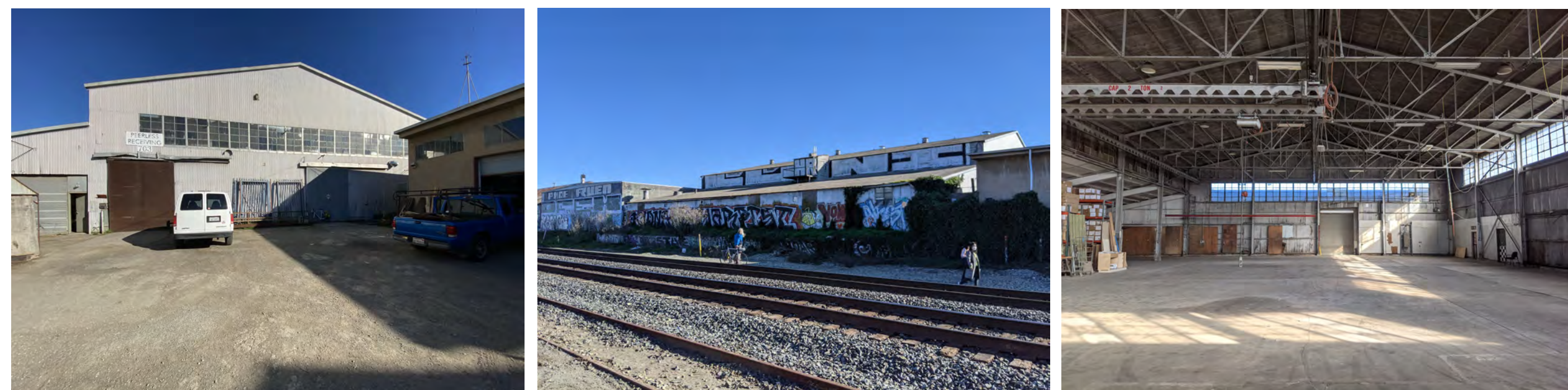
SOUTH FACADE FACING INTERIOR LOT
