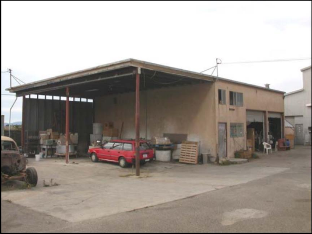
Front view, looking northwest.
