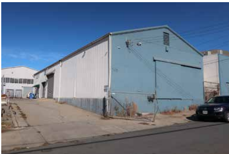
Fig.4 – 705 Bancroft Way, west side and front (looking north from Bancroft)
