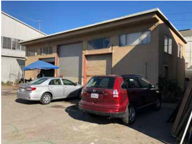
Fig.5 – 705A Bancroft Way, west (front) and south side (looking northeast from site)
