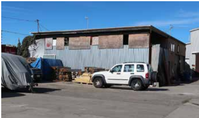
Fig.3 - 701 Bancroft Way, south side (looking north from Bancroft)
