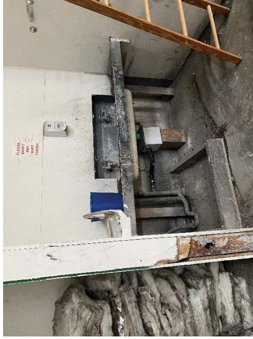
Photo 15: Wash area of the former Ironies Fabrication building.
