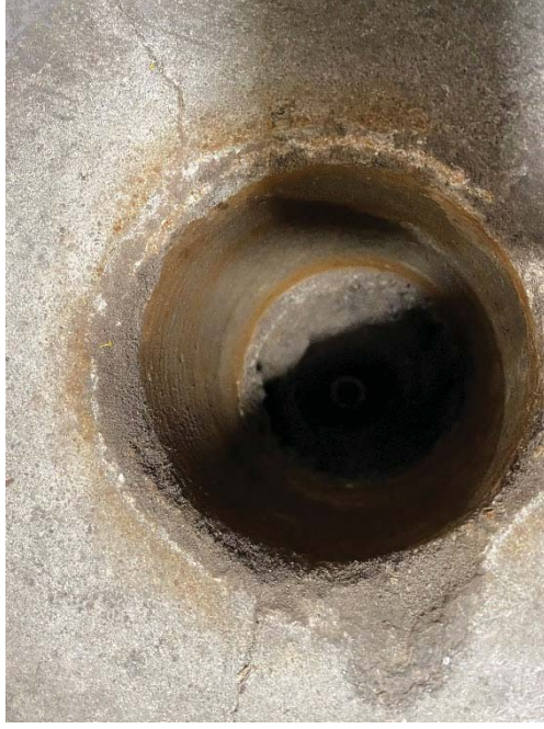
Photo 21: Piezometer located in the former Peerless Electric area of the current WINE.COM warehouse.
