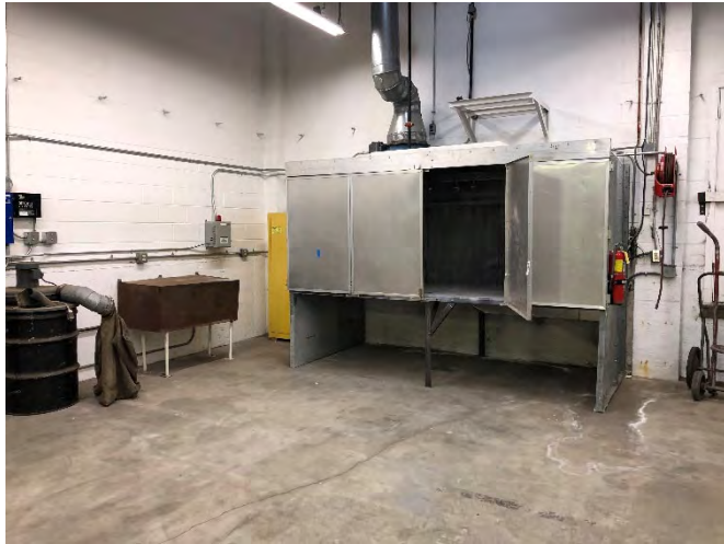
Photo 17: Former laboratory equipment and empty flammable material cabinet located in the 2246 Fifth Street warehouse.
