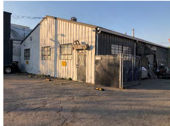
Photo 8: 2216 Fifth Street building.
