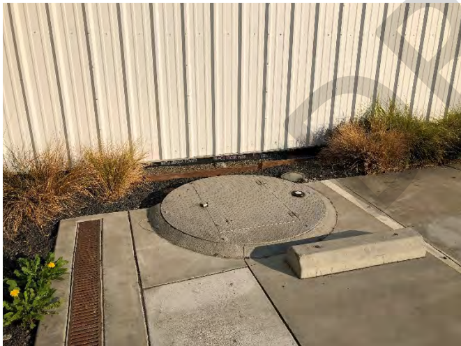
Photo 19: Sump located in the northwest corner of the former Acuity Brands Lighting parking lot.
