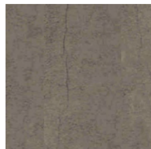
INTEGRAL COLOR STUCCO STEEL HARD TROWEL FINISH
