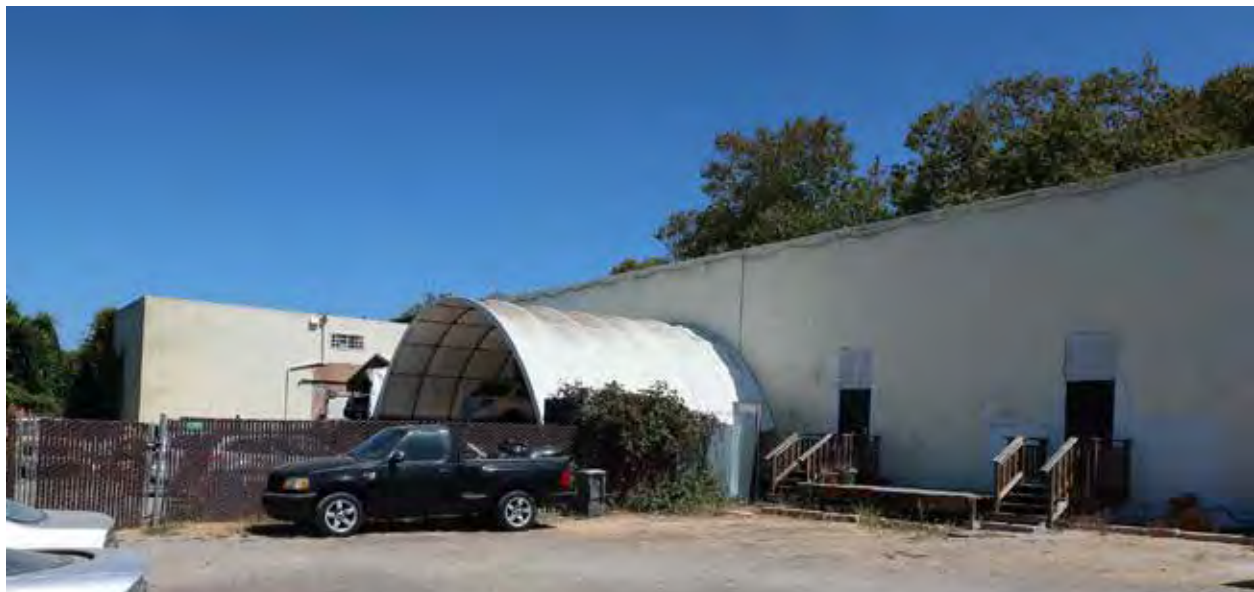
Fig.4 – 2136-2154 San Pablo Ave., Rear (looking north)
