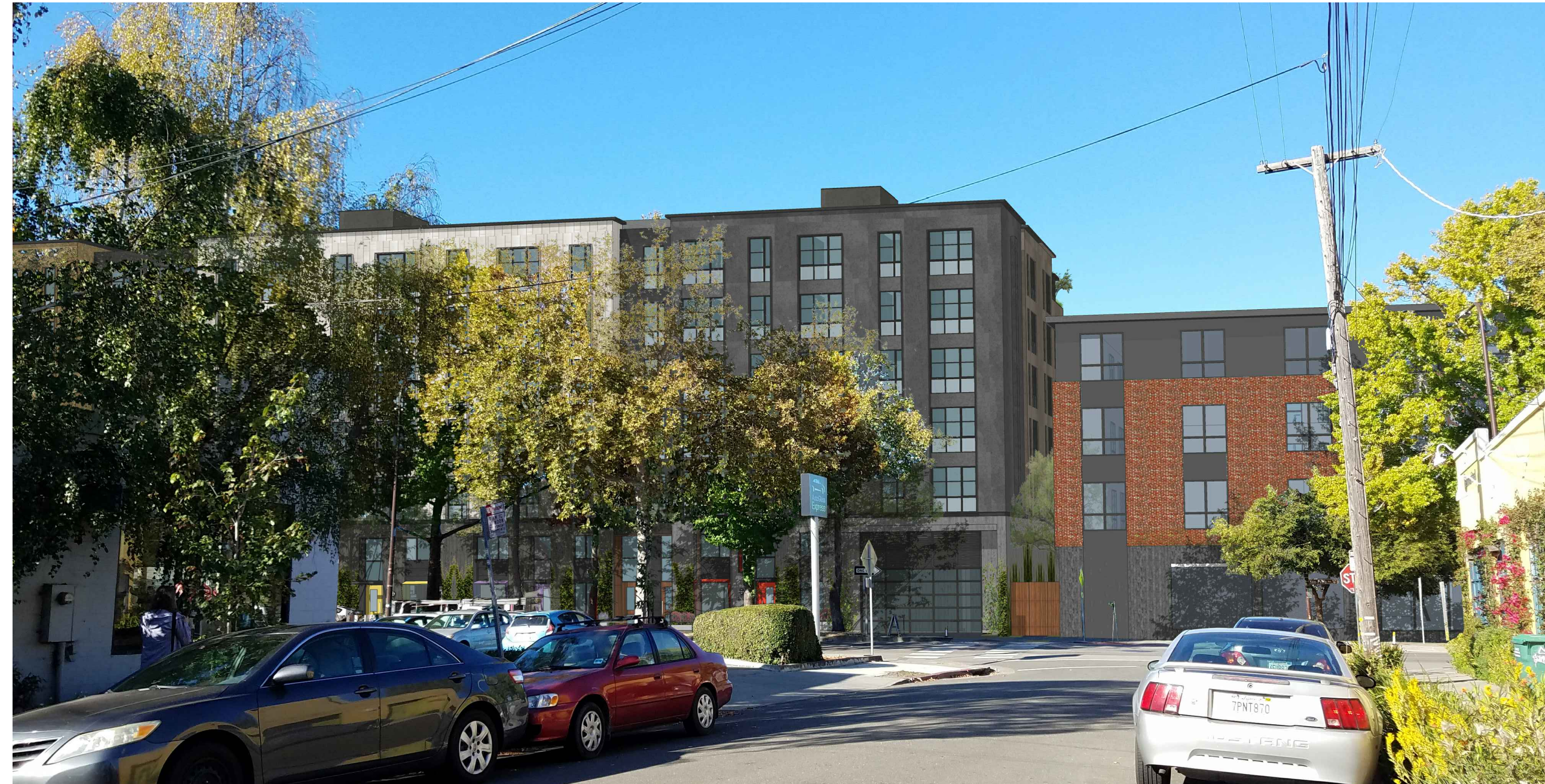
2 - COWPER LOOKING WEST - AFTER
