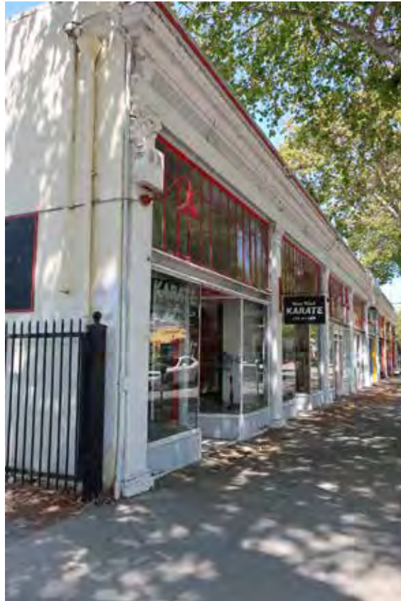
Fig.3 – 2136-2154 San Pablo Ave., front (looking north)
