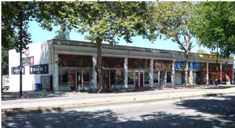
Fig.1 – 2136-2154 San Pablo Ave., front view (looking west)
