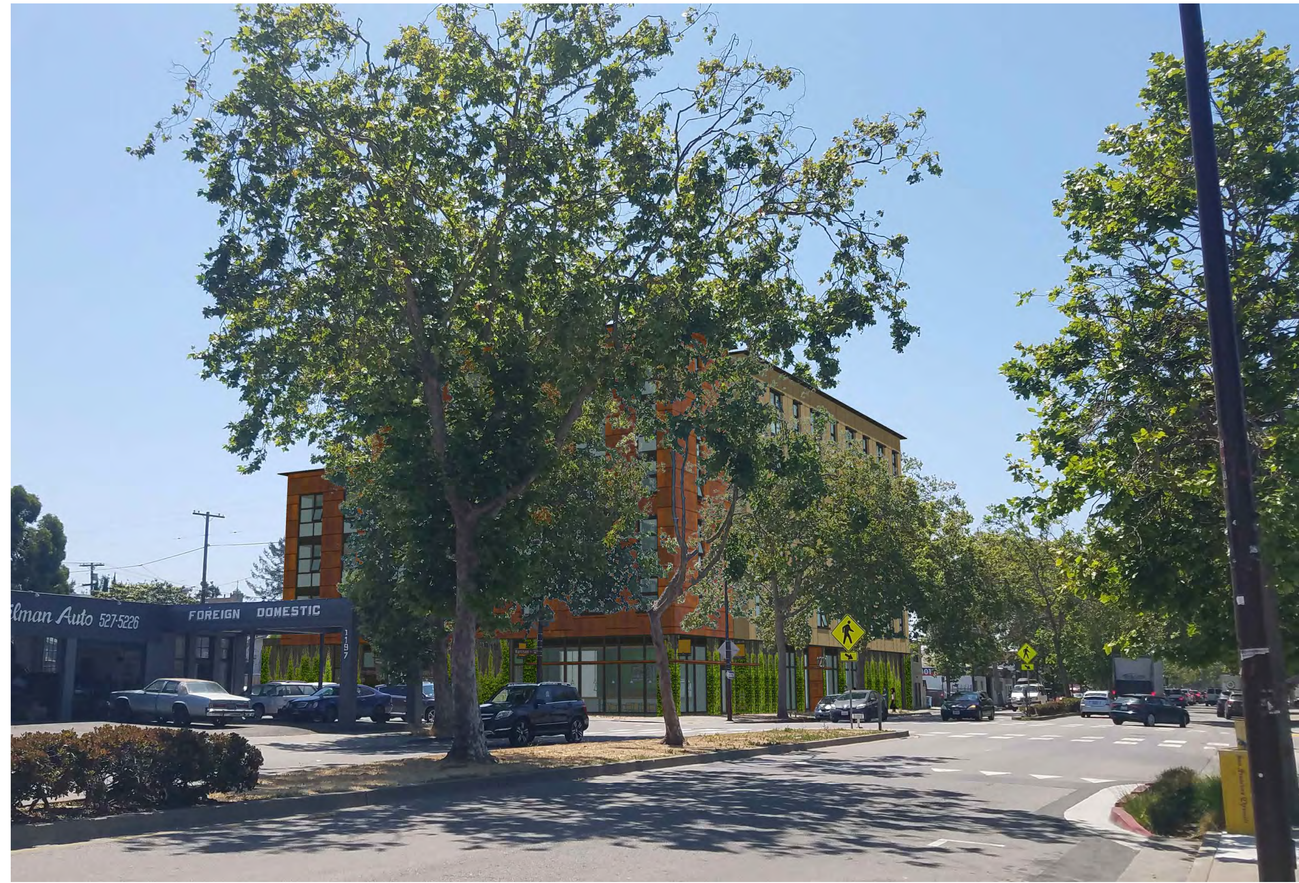
2 SAN PABLO LOOKING SOUTH - AFTER
