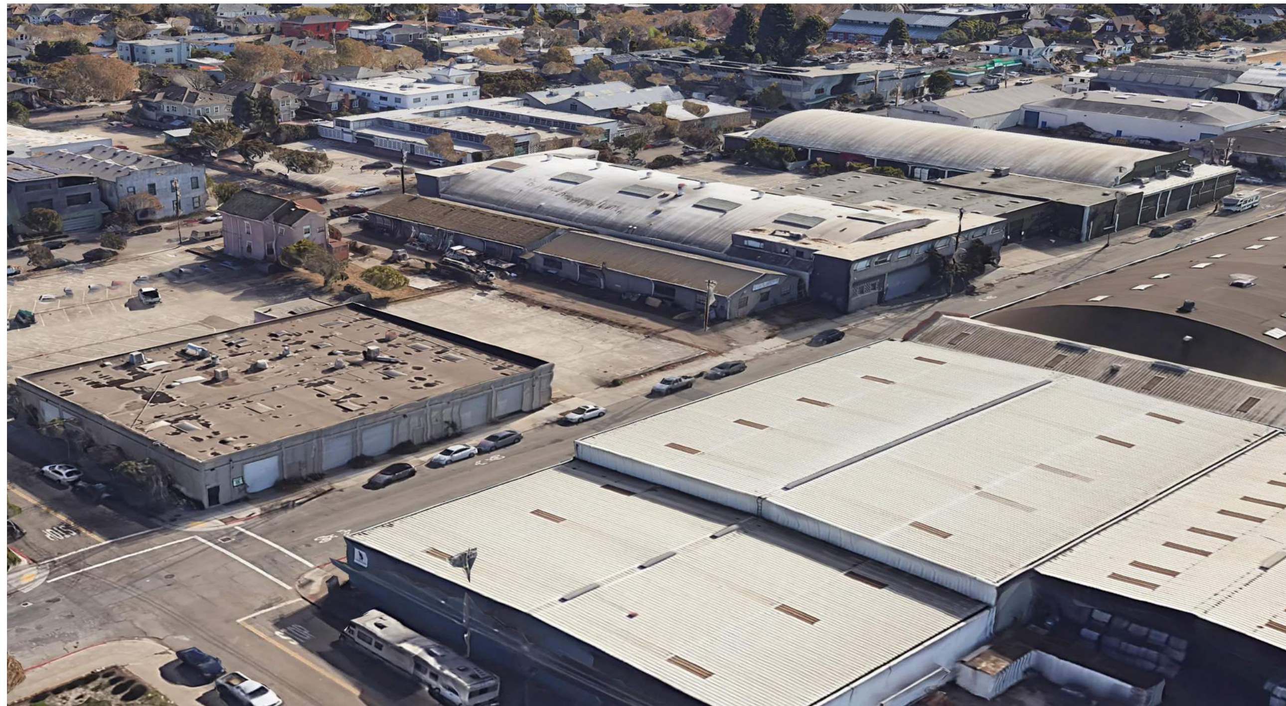
EXISTING AERIAL VIEW FROM NORTHWEST
