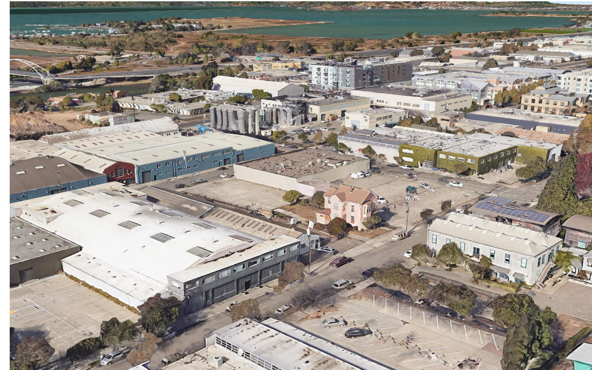
EXISTING AERIAL VIEW FROM SOUTHEAST
