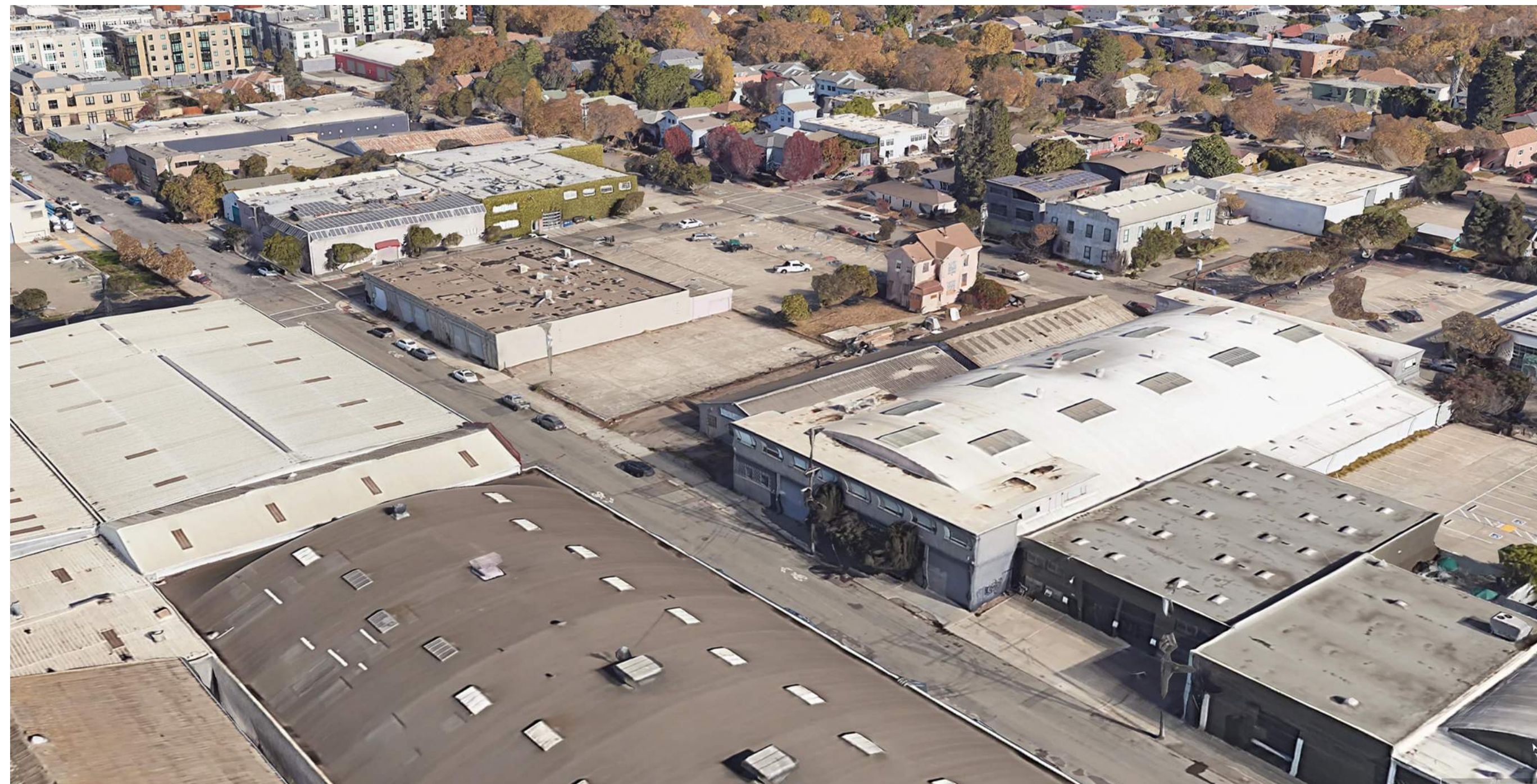
EXISTING AERIAL VIEW FROM SOUTHWEST
