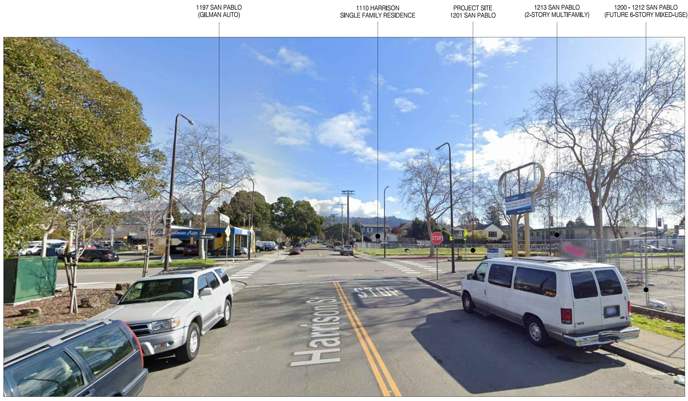
4 - VIEW FROM HARRISON LOOKING EAST
