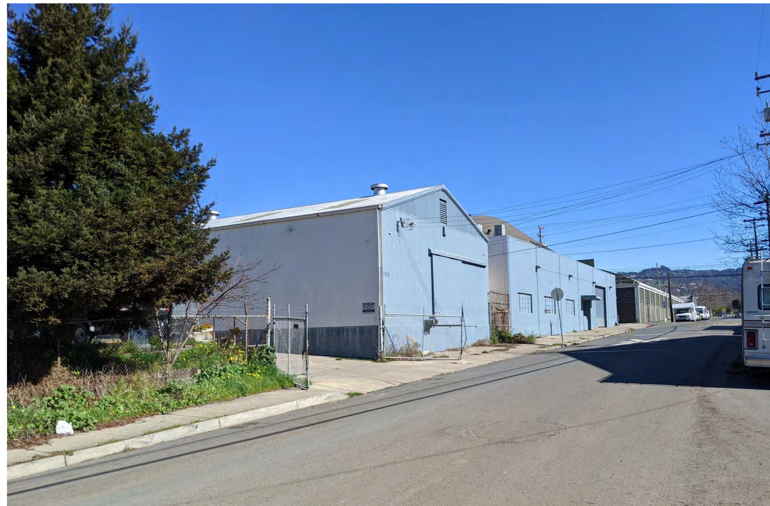
VIEW FROM BANCROFT WAY: EXISTING
