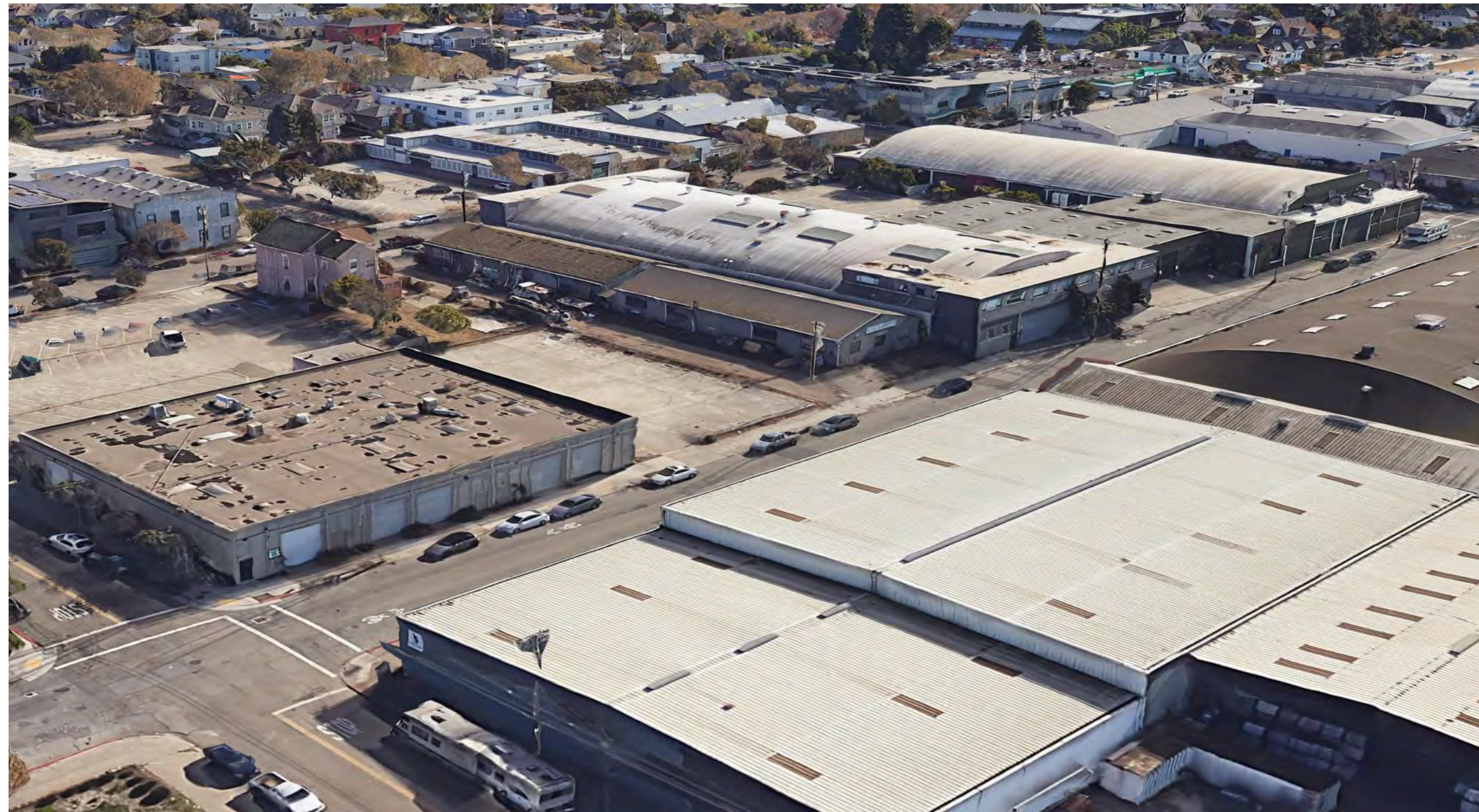
EXISTING AERIAL VIEW FROM NORTHWEST
