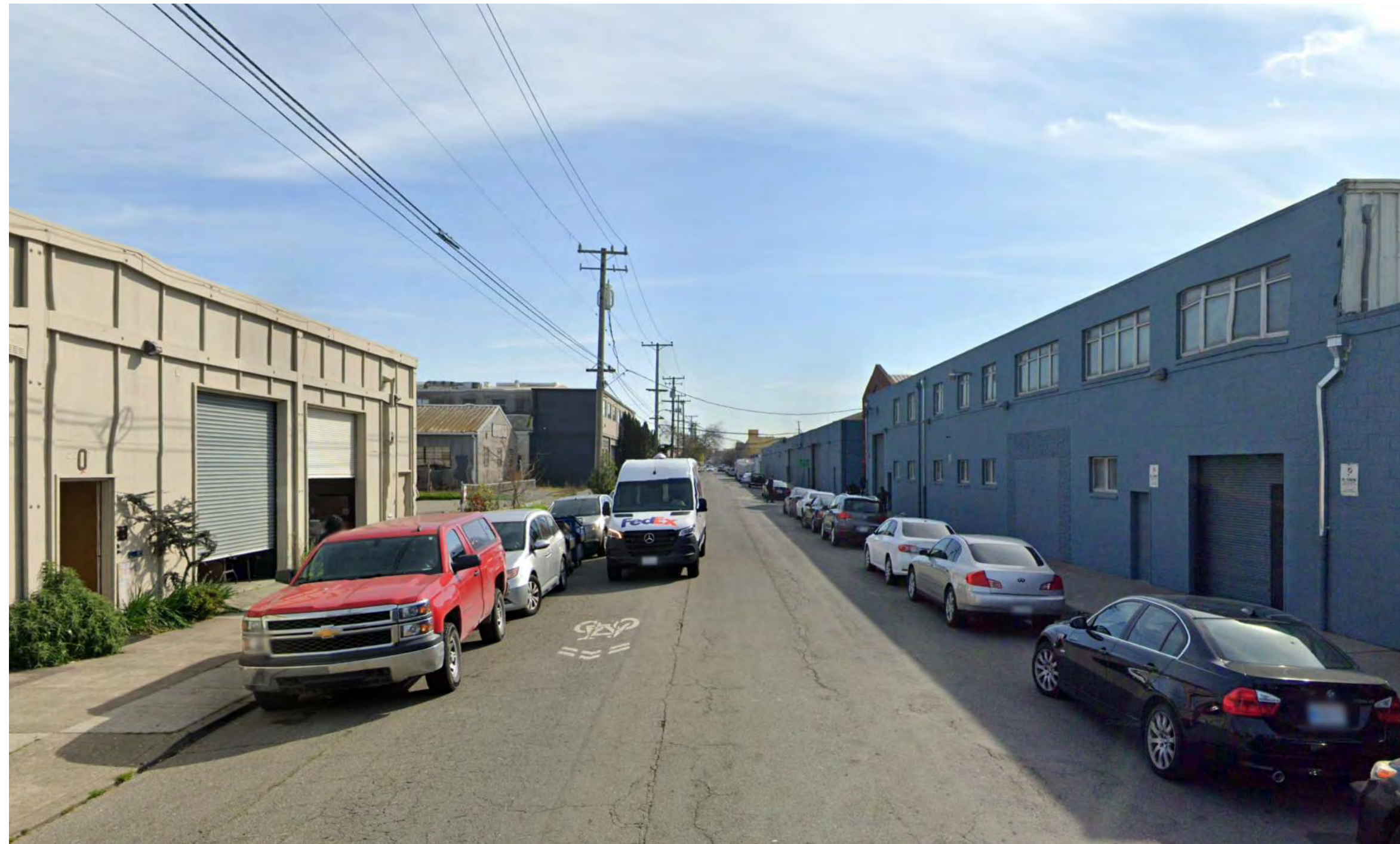
EXISTING VIEW ALONG THE FOURTH STREET - FROM NORTH
