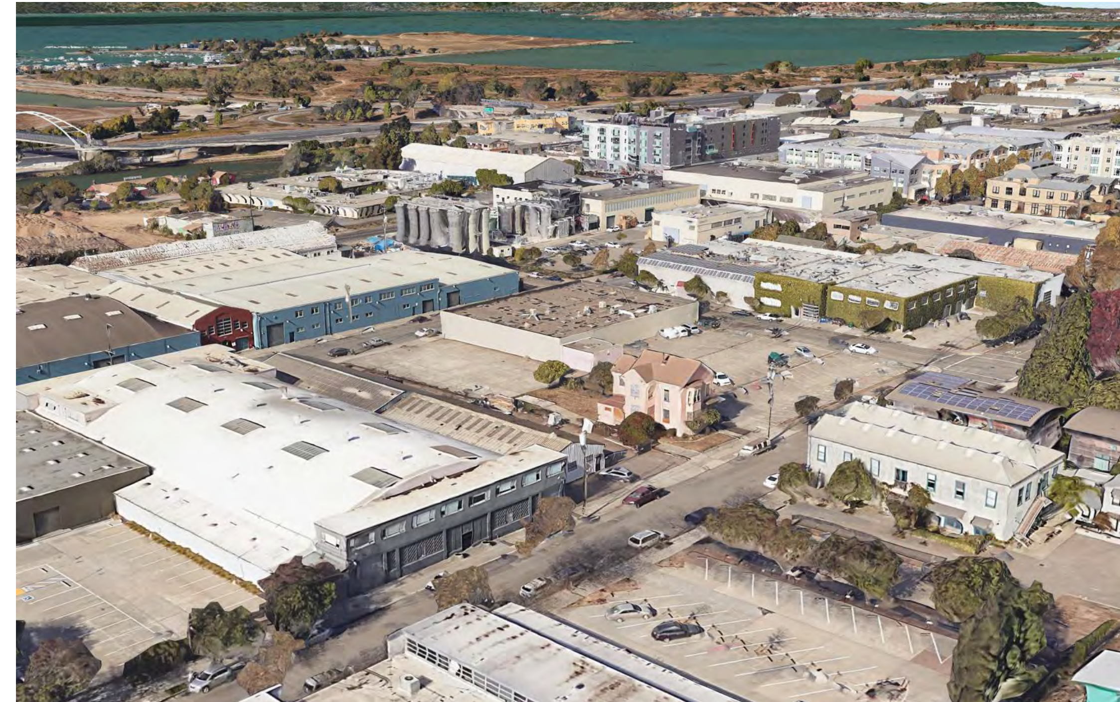
EXISTING AERIAL VIEW FROM SOUTHEAST
