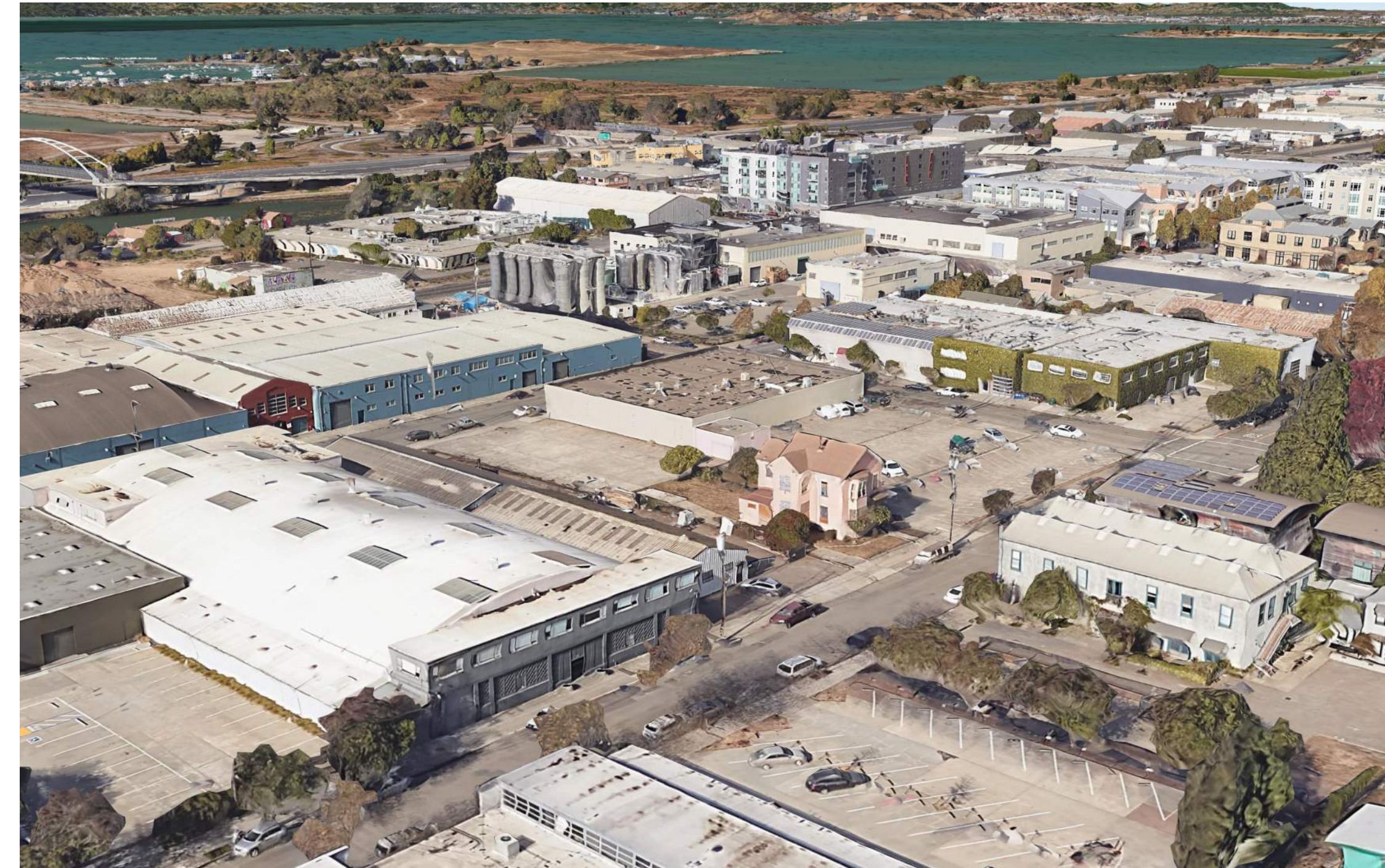
EXISTING AERIAL VIEW FROM SOUTHEAST
