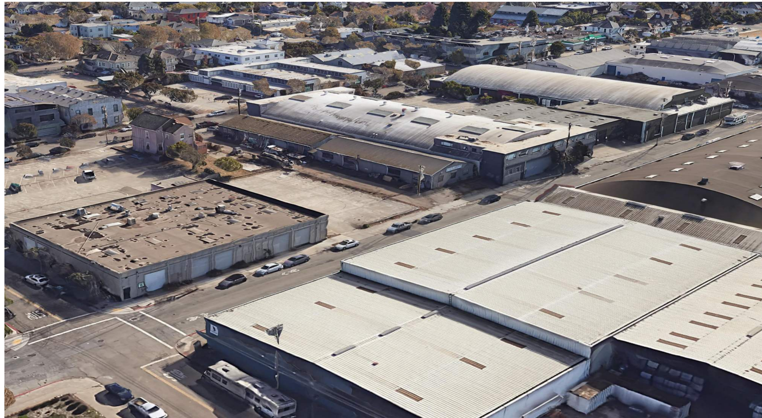
EXISTING AERIAL VIEW FROM NORTHWEST
