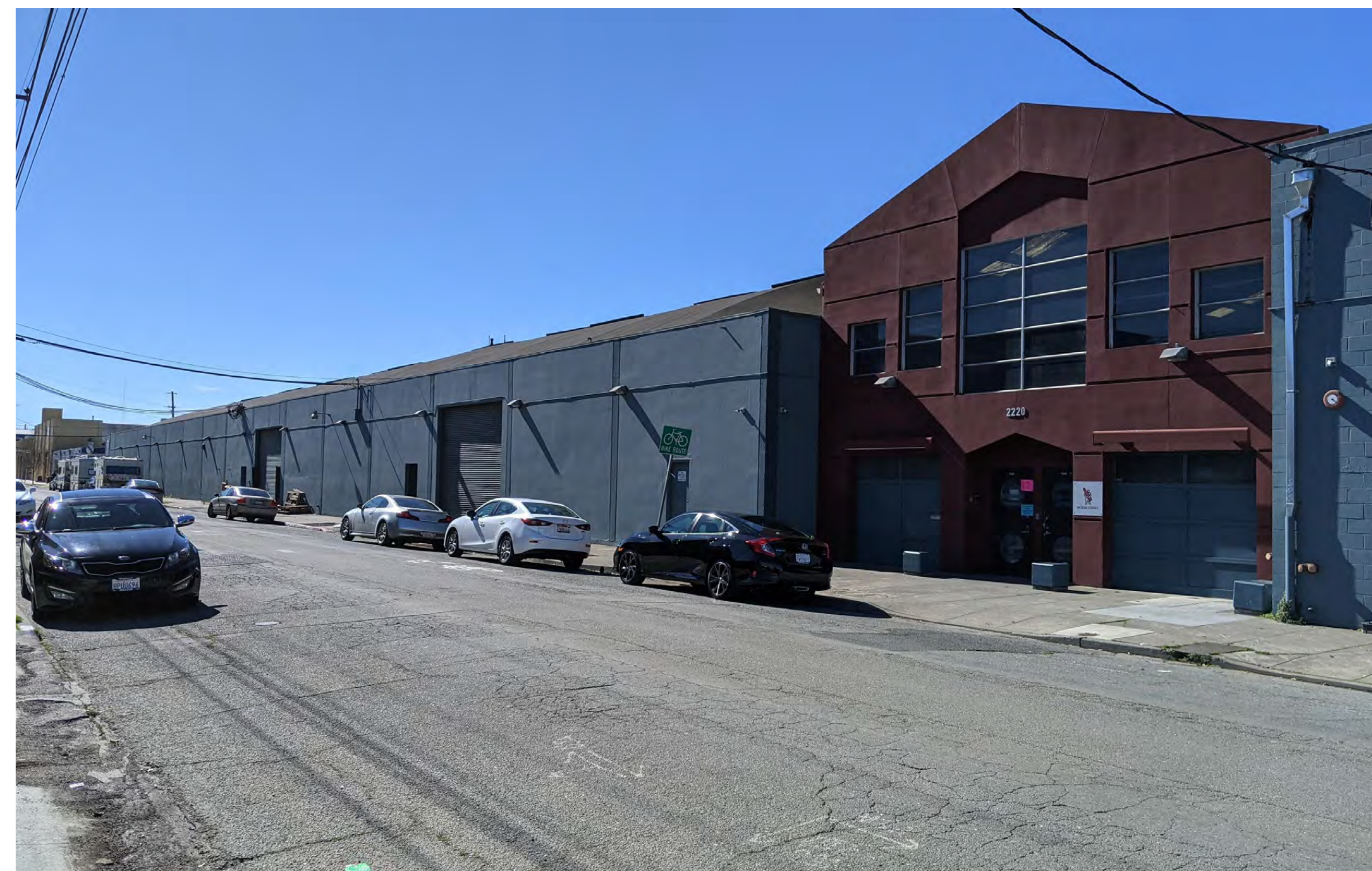
VIEW FROM 4TH STREET: EXISTING
