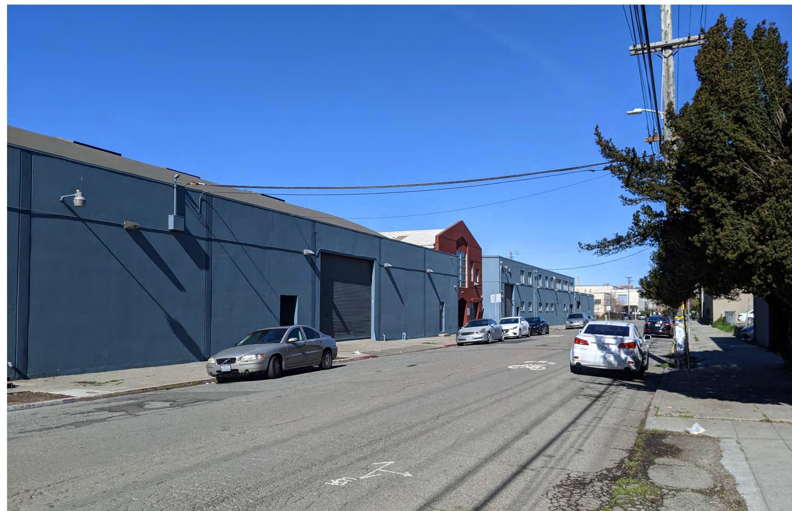
VIEW FROM 4TH STREET: EXISTING
