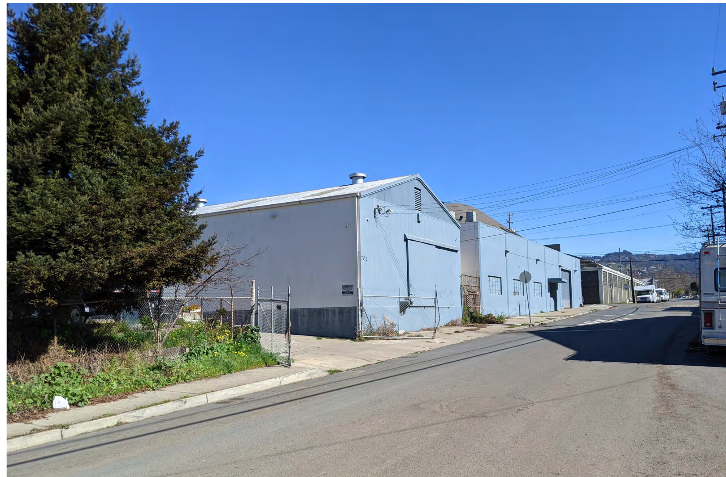
VIEW FROM BANCROFT WAY: EXISTING
