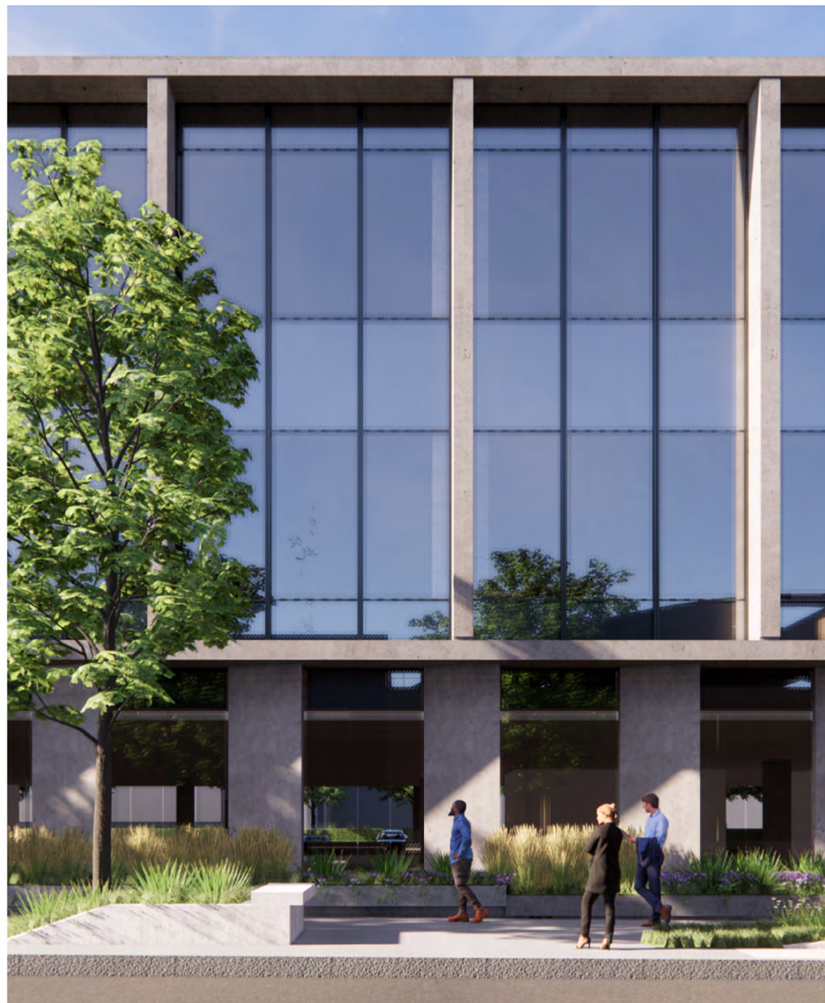
EXTERIOR VIEW AT TYPICAL FACADE (4TH STREET)
