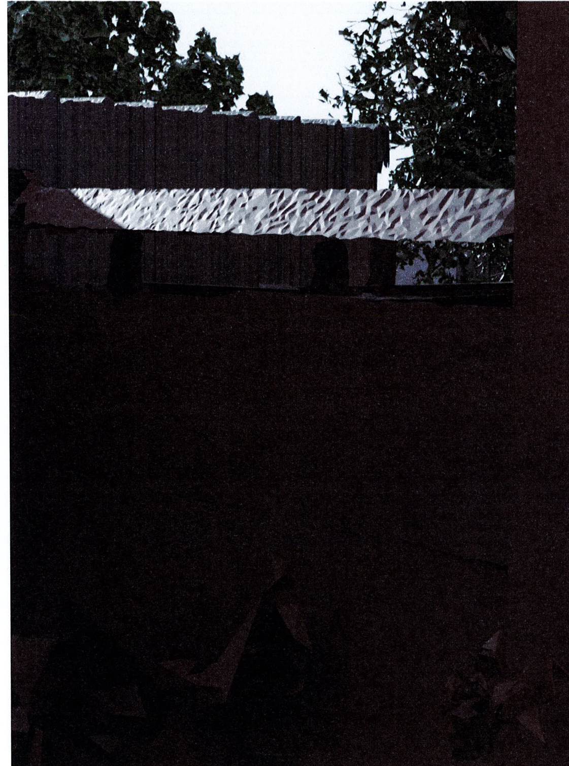
Roof overhang removed
