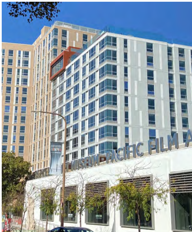
LEFT New Marriott Hotel in Downtown Berkeley
