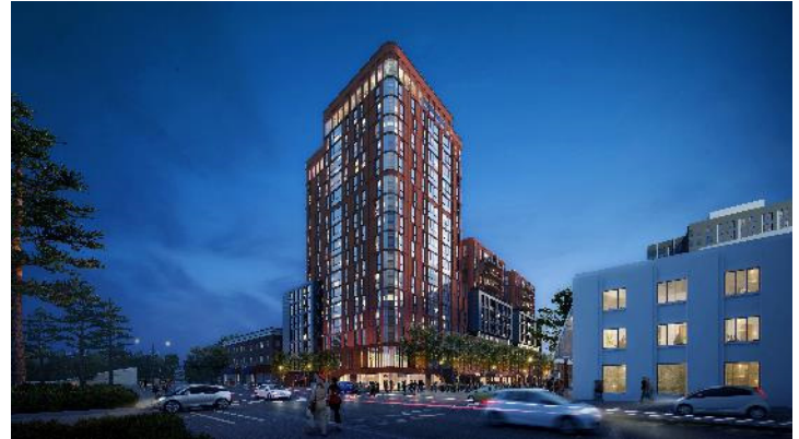
The location of the tower at the Oxford/Center highlights the connection between Downtown and UC Berkeley campus.
