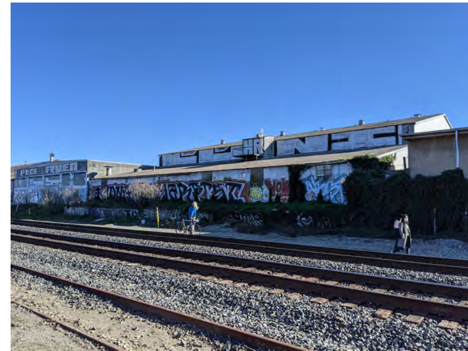
WEST FACADE ALONG RAILROAD
