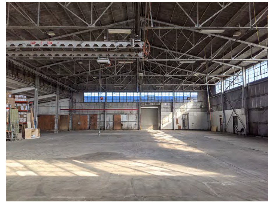
INTERIOR STRUCTURAL FRAME
