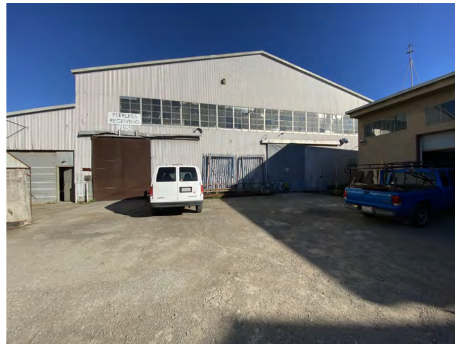
SOUTH FACADE FACING INTERIOR LOT
