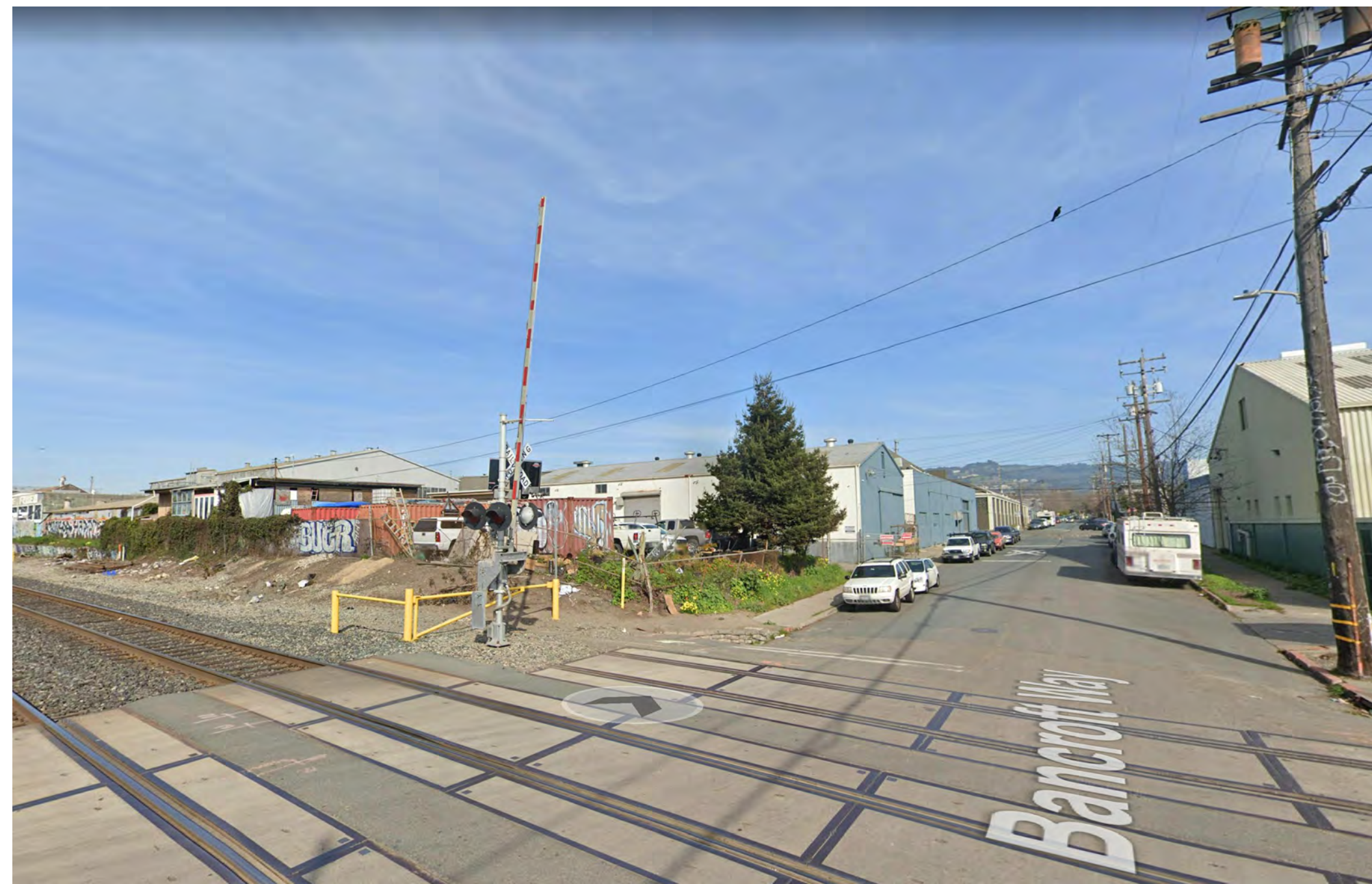
VIEW FROM RAILROAD CROSSING: EXISTING
