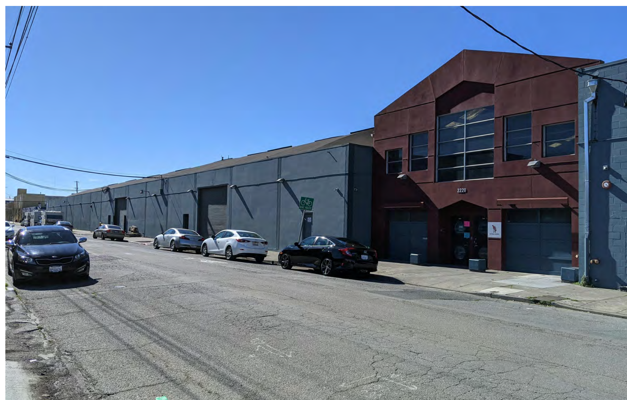
VIEW FROM 4TH STREET: EXISTING
