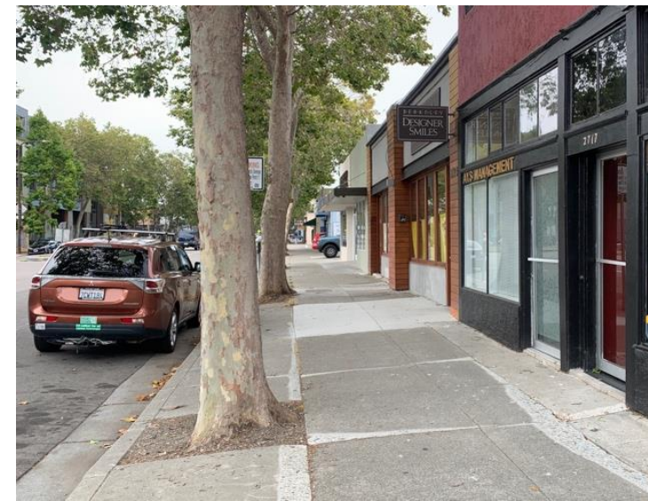
Sidewalks in many locations in need of maintenance
