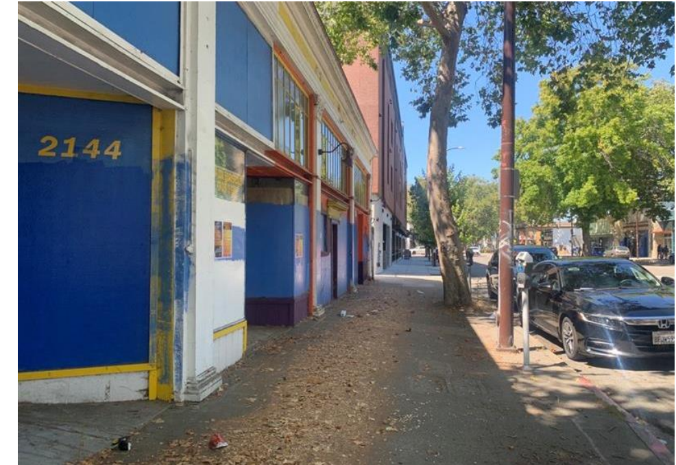
Vacant Storefront. Source: CD+A, 2023
