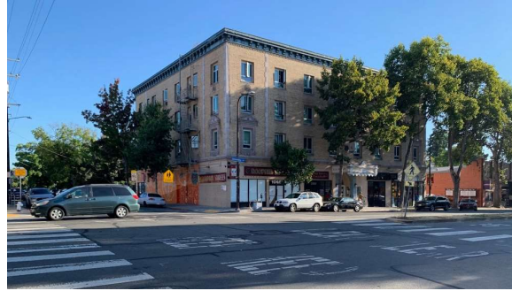
University intersection looking northeast.
