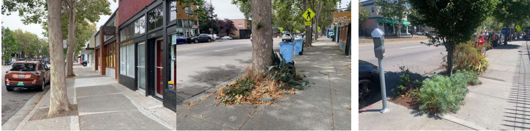
Figure 23. The condition of tree wells varies throughout the corridor.
