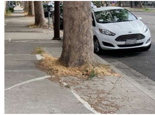
Figure 5.21 Tree on San Pablo Avenue Overgrowing a 3-Foot by 3-Foot Tree Well. Photo by CD+A
