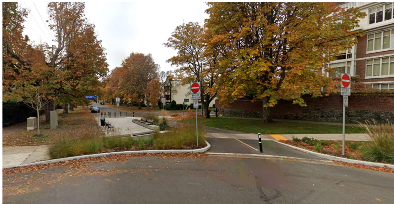
Figure 5.35 Street Closed to Vehicles and Converted into a Plaza With Bicycle and Emergency Vehicle Pass-Through, Vancouver Street/ McClure Street, Victoria, BC. Image from Google maps, Nov. 2022.
