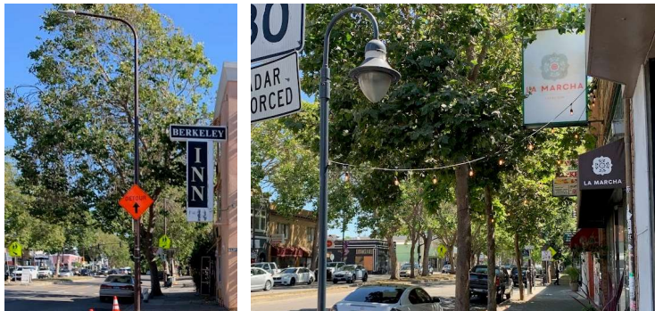
Figure 24. Existing roadway and pedestrian lighting.
