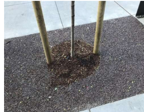
Figure 5.19 Flexible Porous Pavement Downtown Berkeley Tree Well. Photo by CD+A
