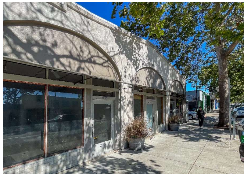
Figure 1.7 Vacant Storefront along San Pablo Avenue. Photo by CD+A. August, 2023
