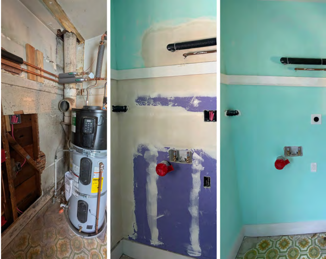
Caption: SolidRock Development Group's progress for Home 19, who received a HPWH, 2:1 ductless heat pump mini split, dryer, and all necessary electrical and plumbing work.
