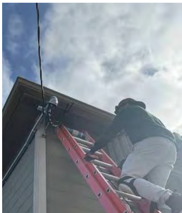
Caption: Micah Electric crew on-site.
