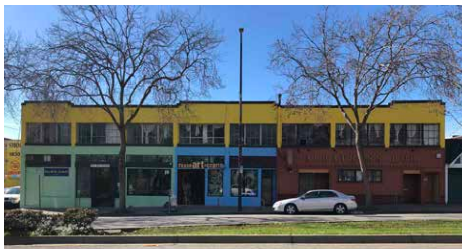
Fig.1 – 1822-1828 San Pablo Ave., front (east)
