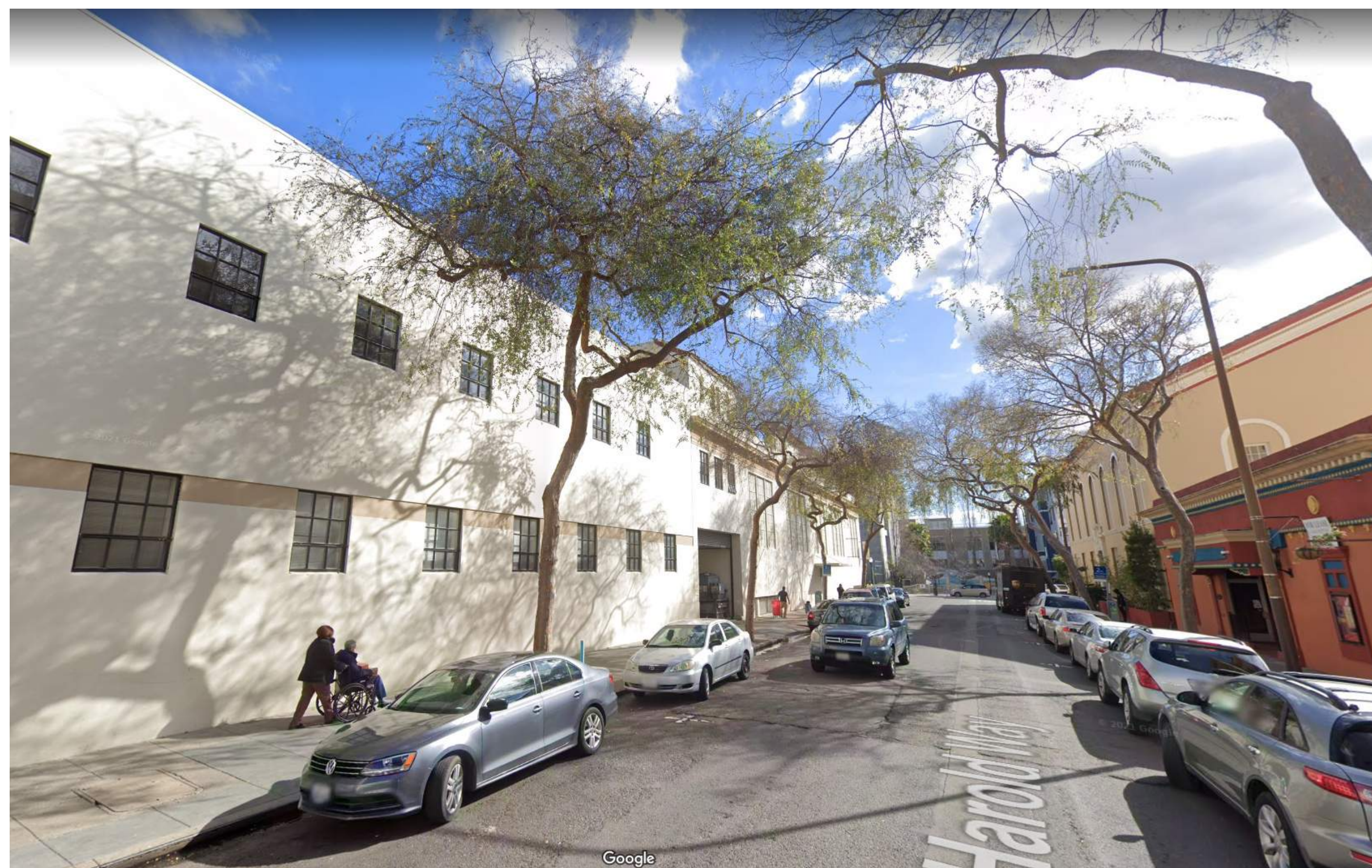
3 SITE PHOTO - HAROLD WAY - LOOKING SOUTH A0-001 12" = 1'-0"
