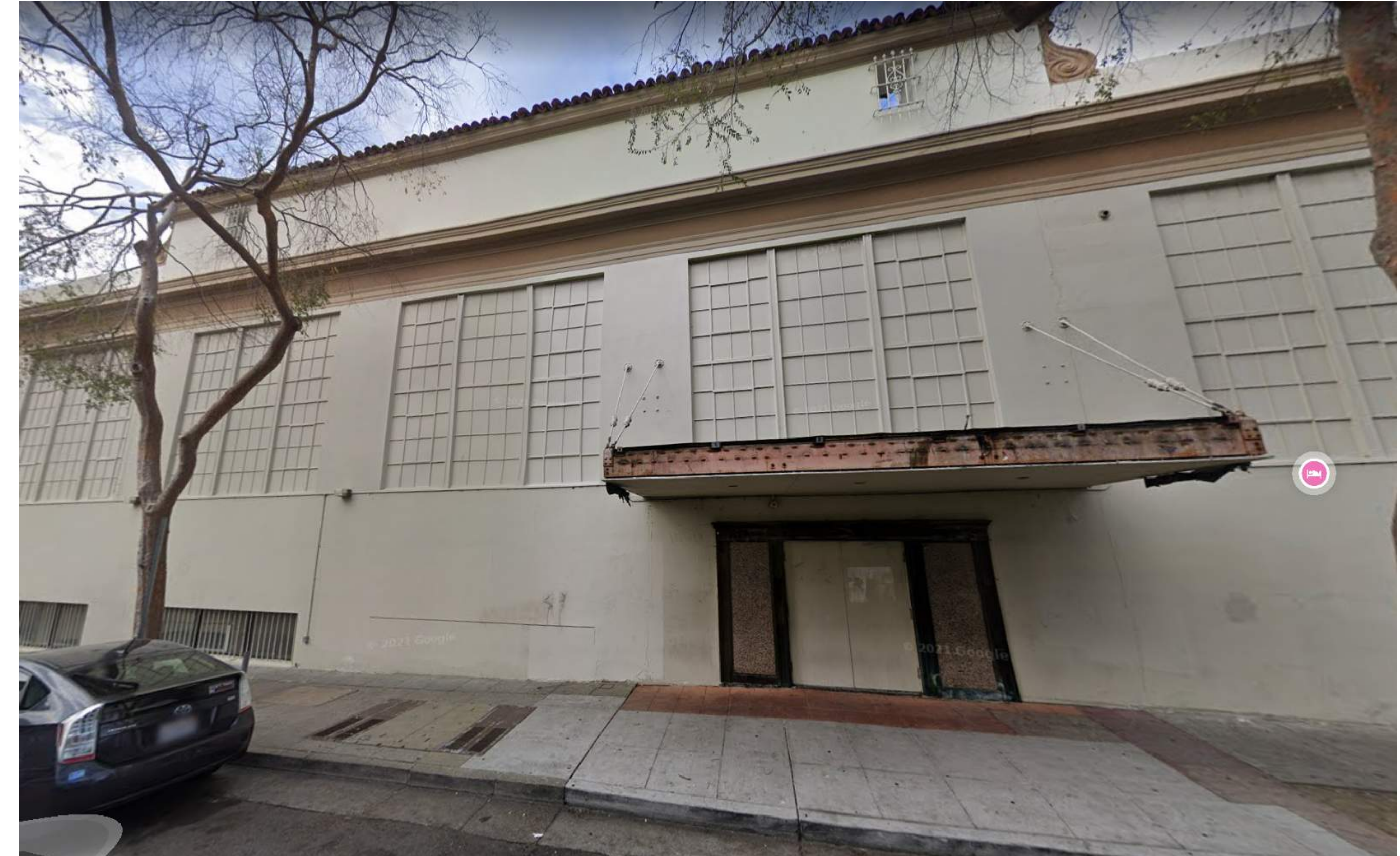
4 SITE PHOTO - KITTREDGE ST FACADE A0-002 12" = 1'-0"
