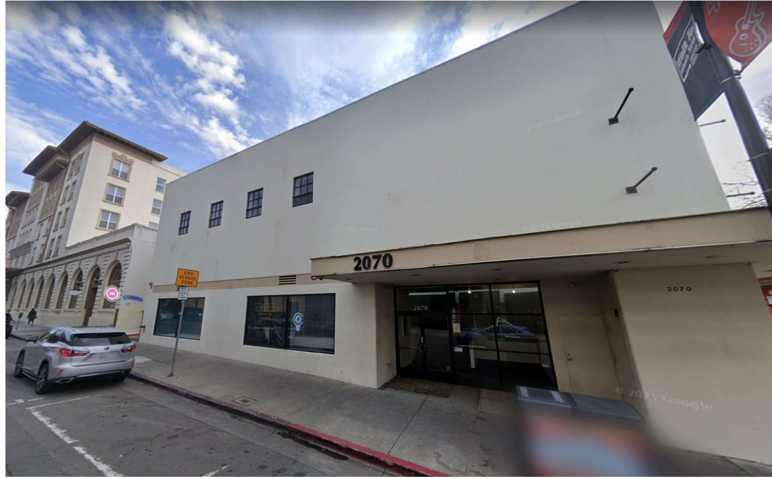
1 SITE PHOTO - ALLSTON WAY FACADE A0-002 12" = 1'-0"
