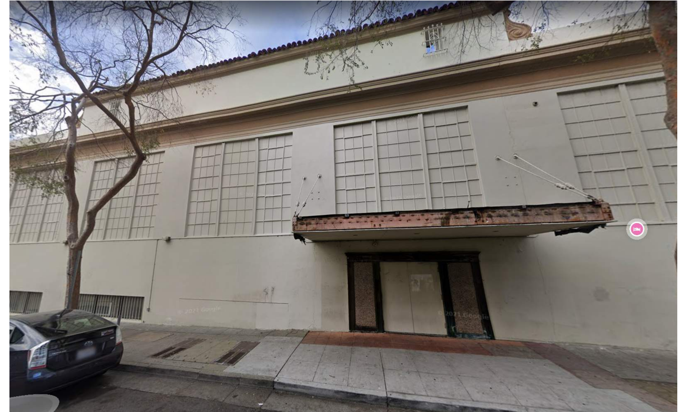
4 SITE PHOTO - KITTREDGE ST FACADE A0-002 12" = 1'-0"
