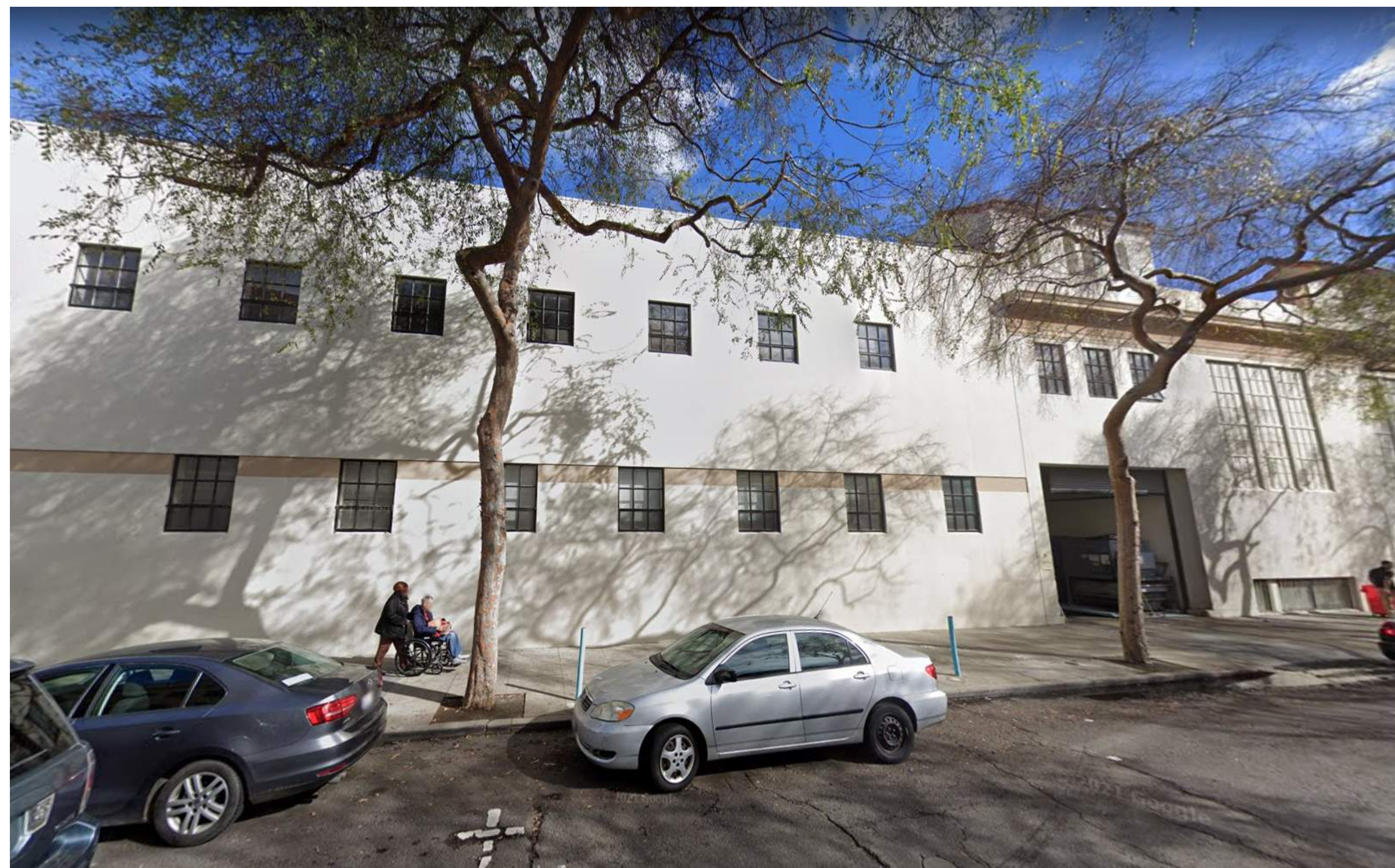
2 SITE PHOTO - HAROLD WAY NORTH FACADE A0-002 12" = 1'-0"
