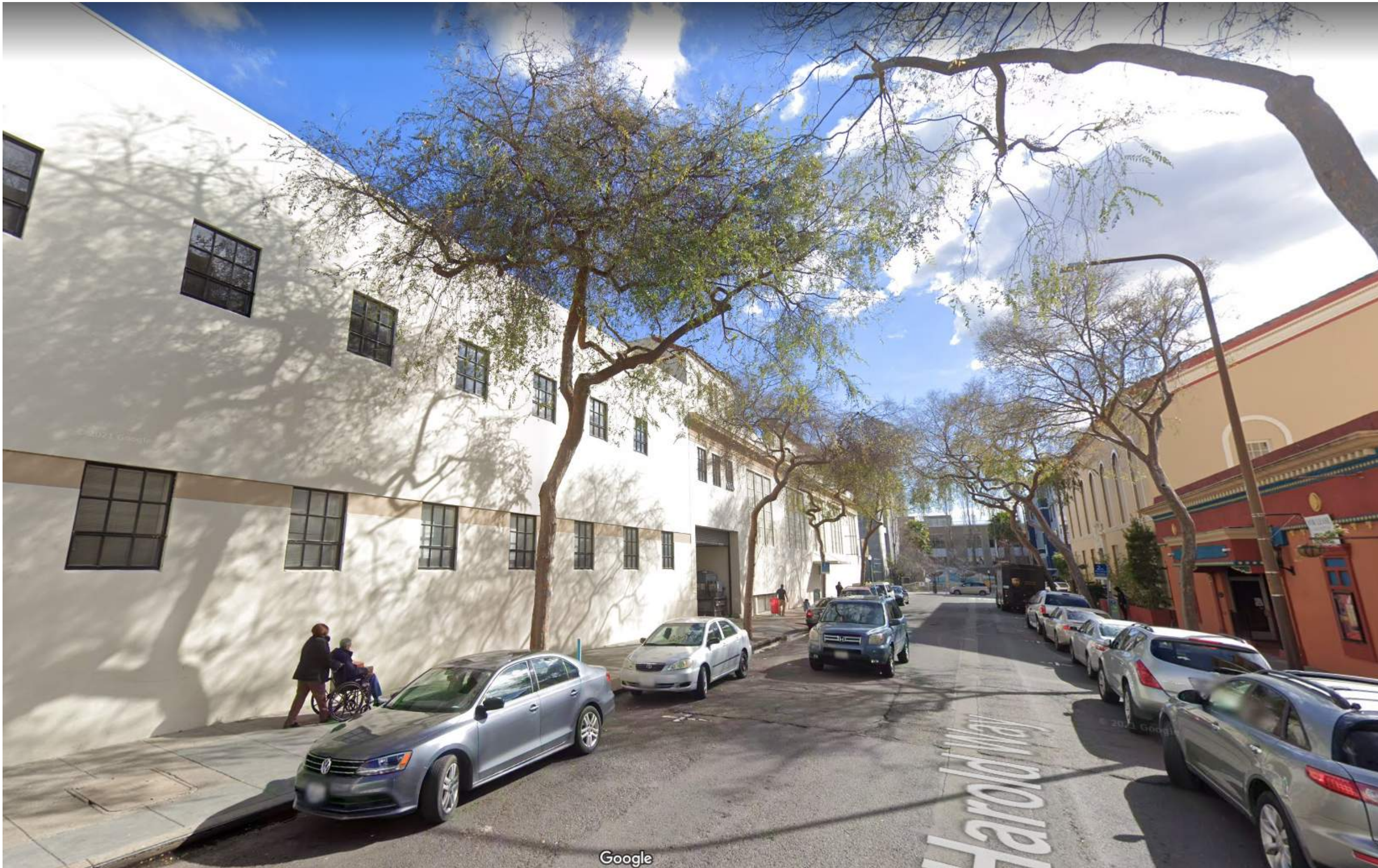
3 SITE PHOTO - HAROLD WAY - LOOKING SOUTH A0-001 12" = 1'-0"
