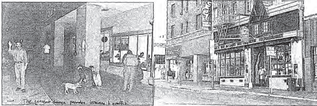
Photo 16. Cambridge Apartments, prior to groundfloor façade rehabilitation.
