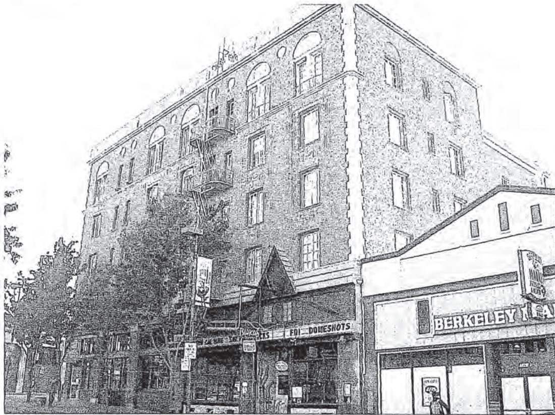
Photo 2. August 2007. The Cambridge Apartments, looking northeast.
